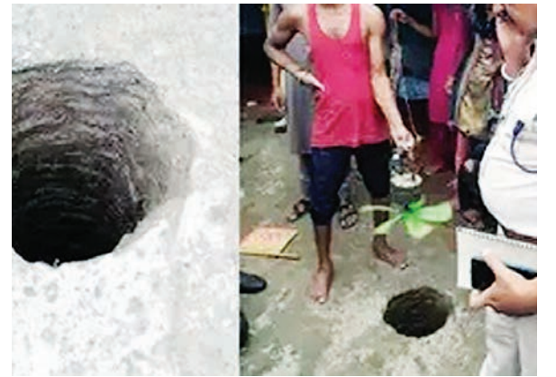
ments started at around 1 p.m. The teams reached the spot and arrangements for oxygen were also made. The rescue operation continued till around 4.30 a.m. on Thursday morning. Excavation started again after putting in place a security cordon. Traffic was stopped by creating a security cordon around the borewell. Big machines are being brought to remove the body from the spot. The biggest problem in the rescue was related to digging because there is a house on one side and a high tension wire above. Officials say that the high tension line will be cut so that the digging machines can work properly.
