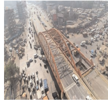
CM Shinde said, "MMRDA is making huge and successful leaps toward infrastructure development and sustainability through a series of ambitious and innovative projects from time to time. This flyover is one of the intuitive projects that are essential in redefining transportation infrastructure in the Mumbai Metropolitan Region (MMR), and I feel elated to have inaugurated
