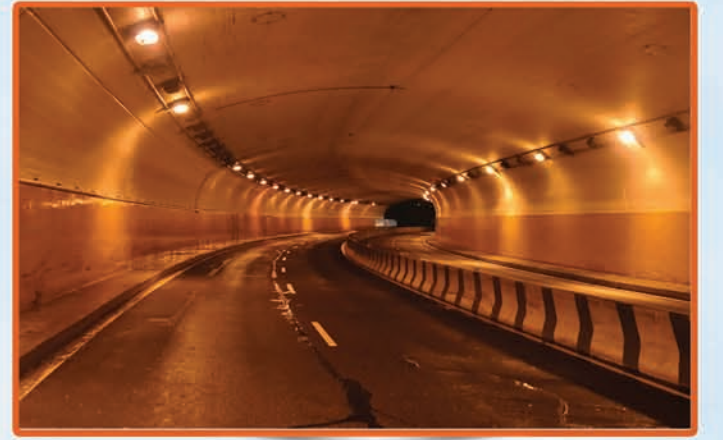
Orange Gate to Marine Drive underground tunnel project
